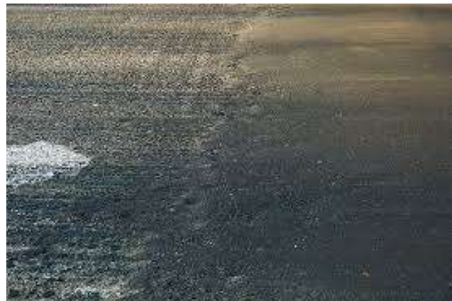
A road displaying rough and smooth pavement textures
