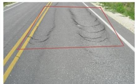
Too High  $\rightarrow \Delta V_2 \geq 5'$   $\rightarrow$  premature cracking, raveling and skipping.
